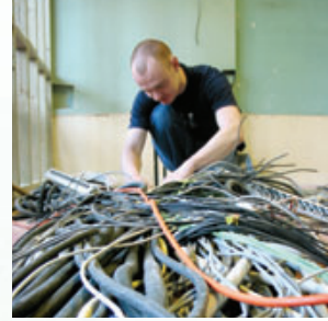
Insufficient planning and use of legacy cabling can run your costs right through the roof.
